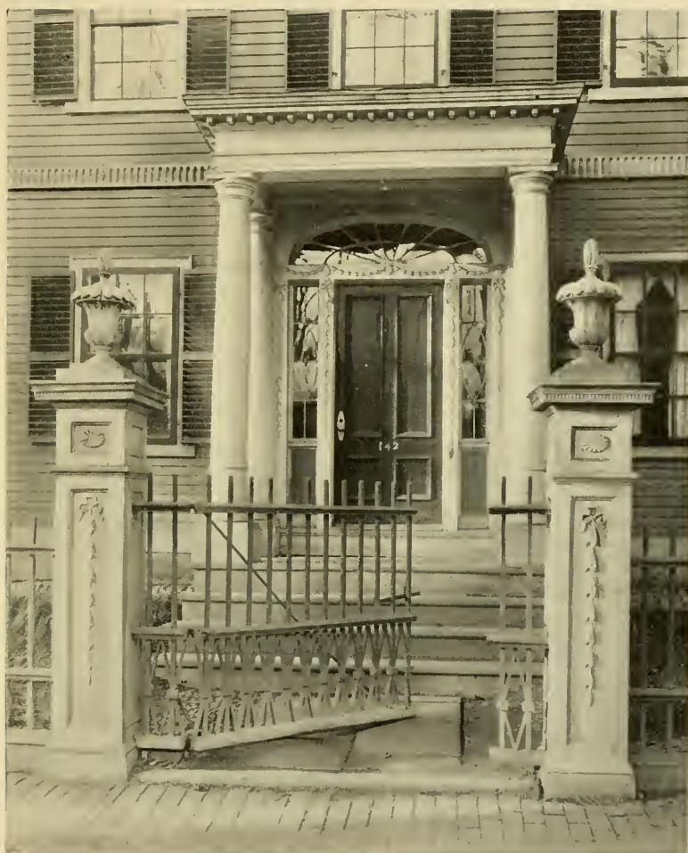
PLATE II. — Doorway, Oliver House, Salem, Mass. Built in 1802.
